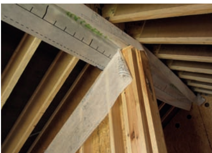
Connection between partition and ridge dial. The continuity of the air barrier is ensured by a suspense membrane (illustration, magazine CSTC -Contact nr. 33 (2012)
