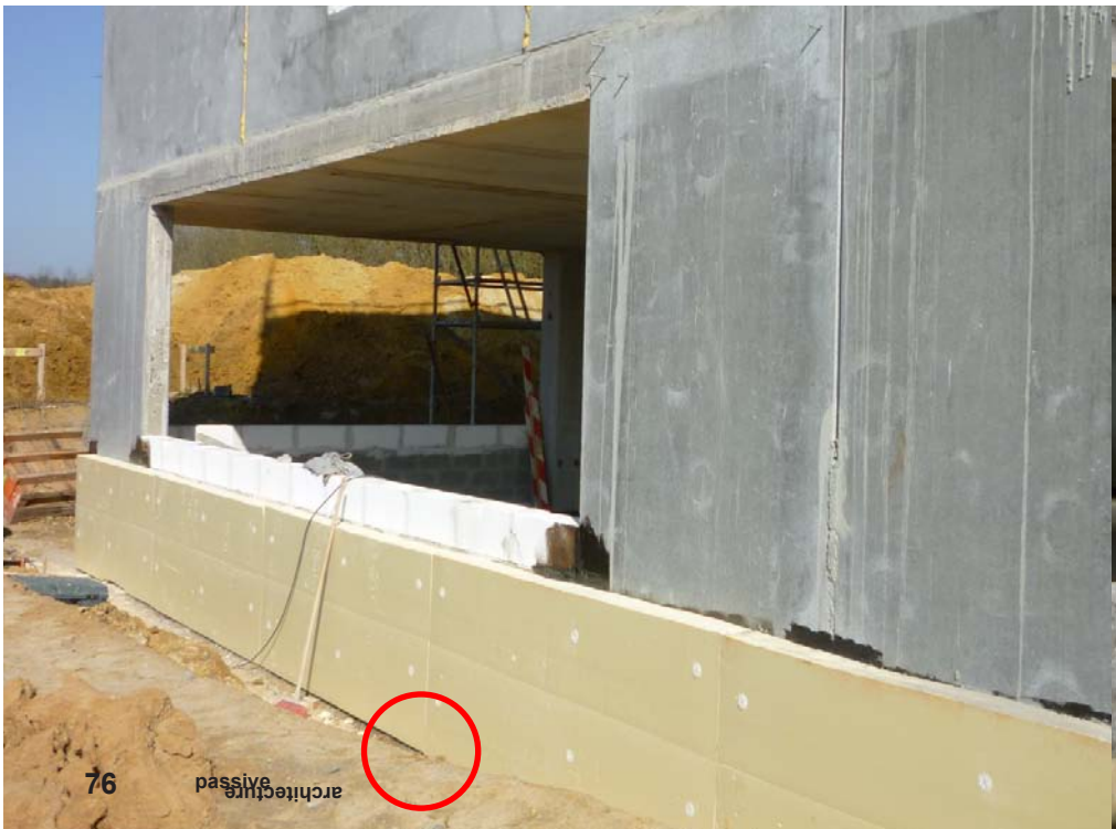
Junction with no insulation block in the brickwork: \Psi=0,27 \text{ W/m.K}
