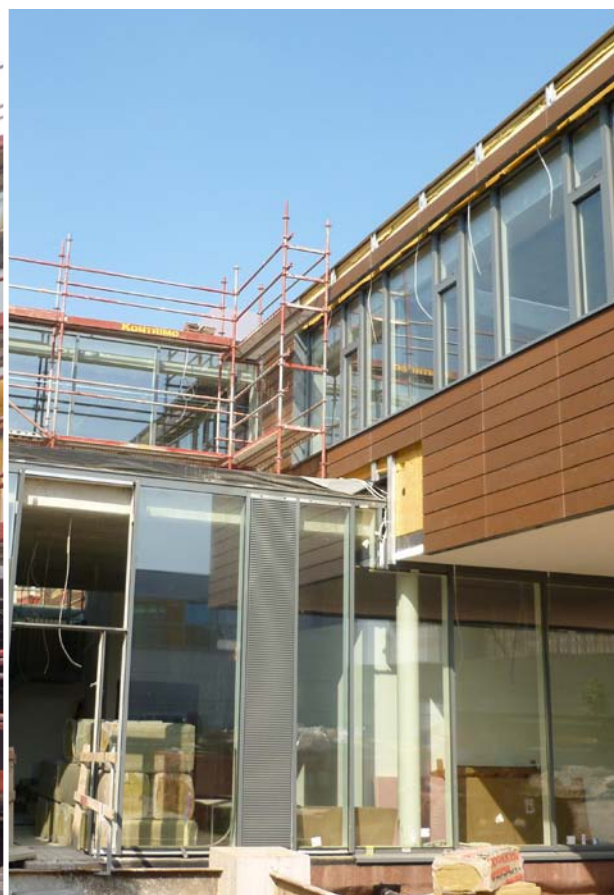
FBZ HQ | Brussels | FBZ | architect: A2M
