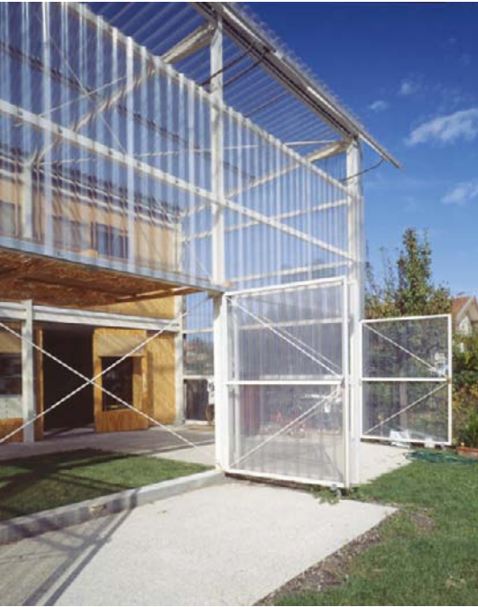
House Latapie | Floirac | private | architect: Lacaton & Vassal
