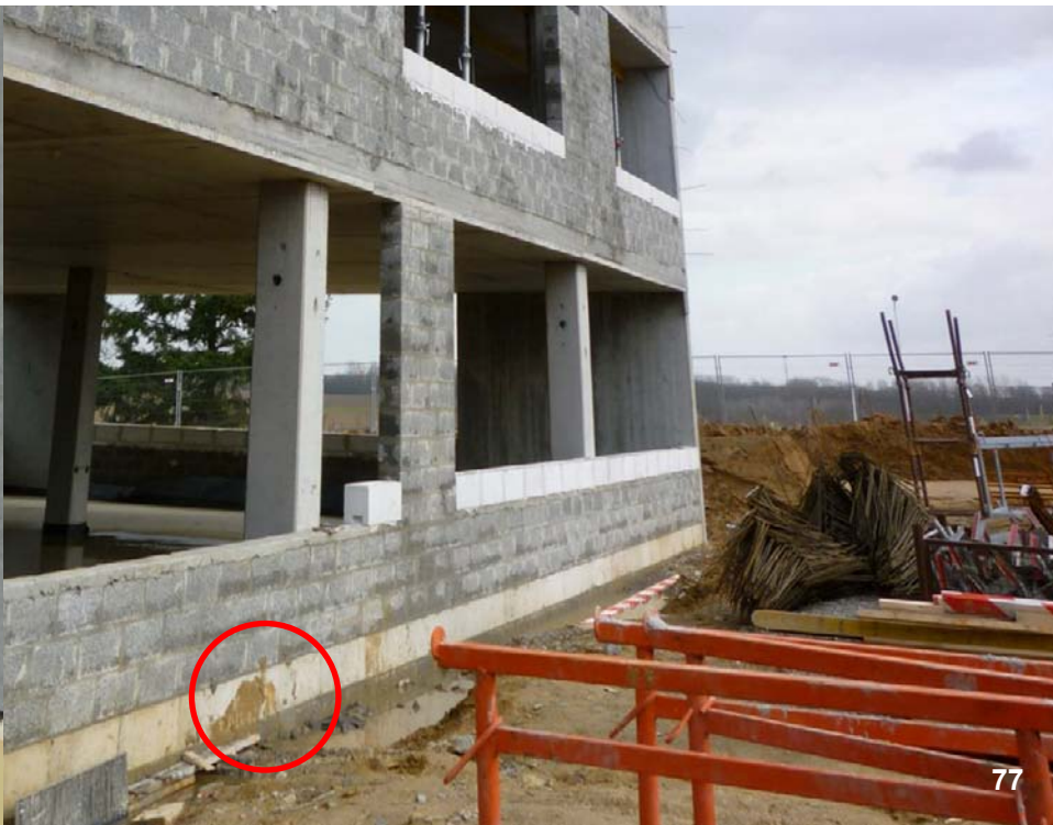
Junction including an insulation block in the brickwork: \Psi = -0,02 \text{ W/m.K}
