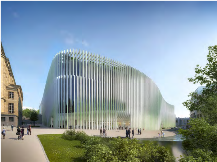
BNP Paribas Fortis Bank Headquarter | Brussels | BNP Paribas Fortis | architect: Baumschlager & Eberle et Styhals & partners
